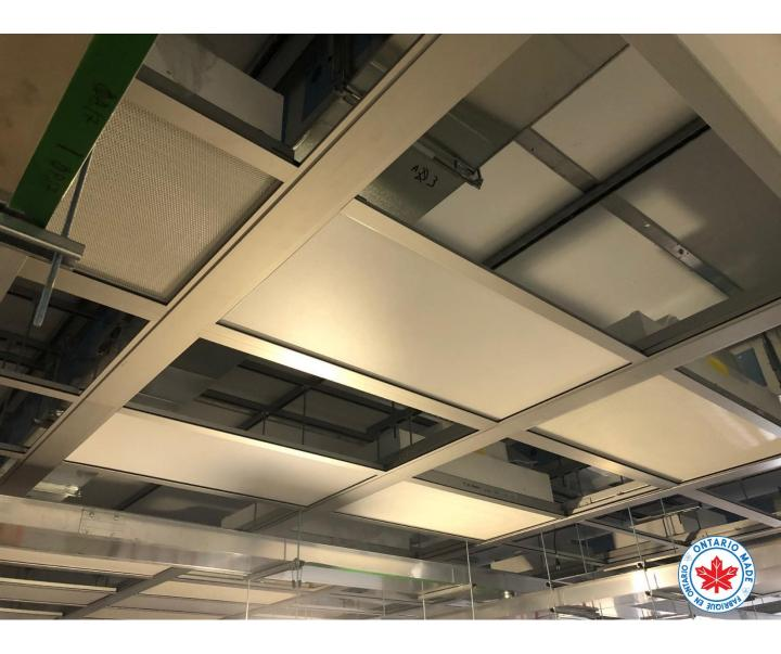
ASI Series 2" ceiling grid systems assist in the ever-changing design needs to create the next generation of social open preengineered all modular design features for general laboratory and cleanroom suspended ceiling applications that can foster team-based research interaction while providing a system design balance of flexibility, ease of equipment placement, and standard solutions for integration of todays advanced technologies and industry compliance standards.
